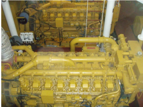
A 16 cylinder diesel generator onboard a ship
